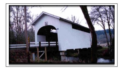
Designed in the typical Howe truss style, this 1929 structure exemplifies all that is romantic about covered bridges. The Harris Bridge is located along a winding gravel road near Wren. It is named after the Harris family who settled out side of Corvallis Oregon in 1890.
