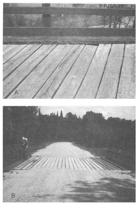
Figure 2-22.- Sawn lumber plank decks (A) in a transverse orientation and (B) in a longitudinal orientation.
