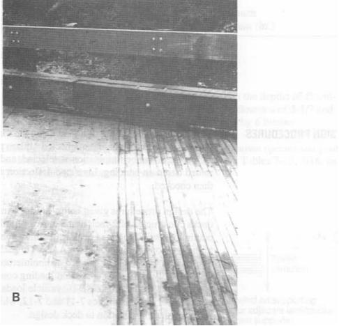
Figure 7-35.—(A) Edge view of a transverse nail-laminated lumber deck. (B) Top view comparison of a nail-laminated lumber deck (right) and glulam deck (left).
