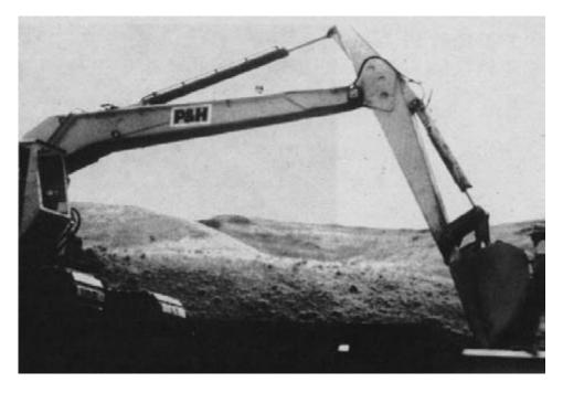
Figure 15-64. - Backhoe pushes panels together after dowels have been aligned. A large timber block was placed across the panel edge to prevent damage from the backhoe bucket.
