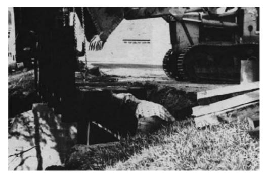
Figure 15-23. - A prefabricated deck panel is lifted onto the abutments. Each panel was prefabricated to fit each bridge.
