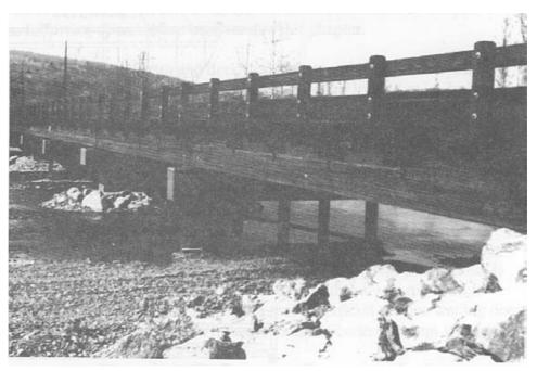
Figure 7-3.- Glulam beam bridge, 290 feet long in Tioga County, New York. This bridge was completely prefabricated in standardized components that were bolted together at the project site (photo courtesy of Weyerhaeuser Co.).
