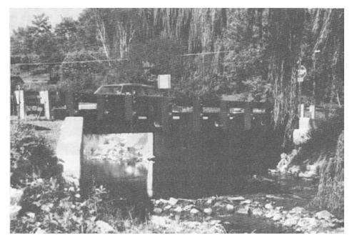
Figure 2-28- Stress-laminated deck bridge built near State College, Pennsylvania, in 1987. The bridge is 28 feet wide and was constructed from 4-inch-wide by 16-inch-deep lumber laminations.
