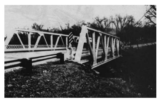
Figure 15-47. - The existing bridge was a steel truss, 96 feet long, with a 26-foot roadway width. The noncomposite concrete deck was supported by steel stringers (WF16 x 50) spaced 4 feet 6 inches on center. The stringers were supported by steel floor beams (WF30 x 116).
