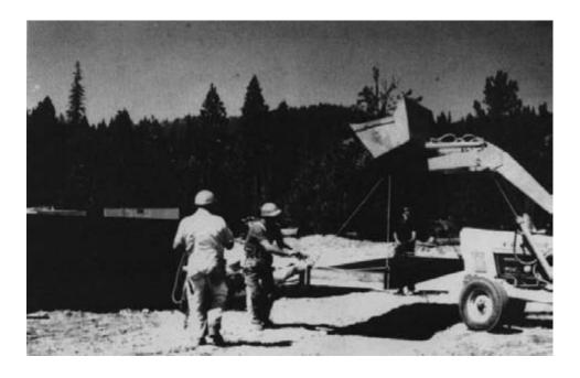
Figure 12-8. - Lifting a glulam deck panel from steel C-brackets that fit over the panel ends.
