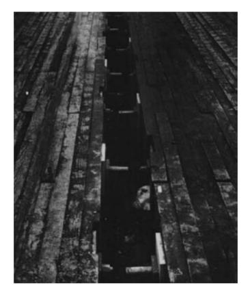
Figure 15-80. - Prestressing rods protruding from the two prefabricated deck panels before connection. The rod opposite each coupler was released and threaded into the coupler. After all couplings were made, the released rods were restressed, causing the deck panels to be stress-laminated together as an integral bridge deck.
