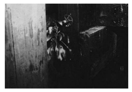
Figure 13-22. - Visual signs of potential deterioration (continued). (E) Plant growth.
