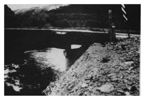
Figure 15-58. - The temporary repair made to the bridge consisted of replacing the approach embankment and lifting the nail-laminated approach span back into position.
