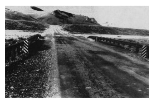
Figure 11-29. - Aggregate wearing surface on a timber bridge deck.
