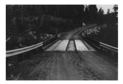
Figure 11-25. - Timber bridge deck with lumber running planks.
