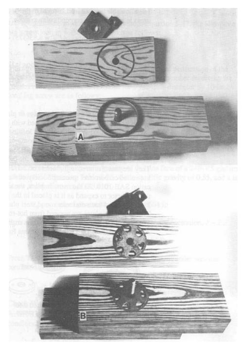
Figure 5-27.- Typical timber connectorjoints: (A) split ring connector between wood members. (B) Shear plates used back-to-back between wood members.
