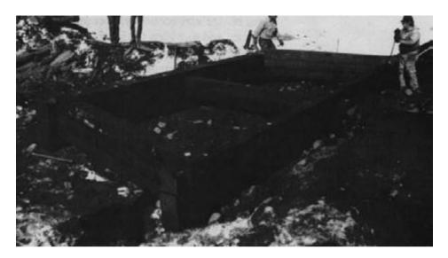
Figure 15-78.-The new crib abutment under construction using precut and creosotetreated Douglas-fir timbers. The only field fabrication involved drilling holes in the timbers for drive spikes used for connections. Such penetration of the protective envelope should have been avoided by drilling before pressure treatment (photo courtesy of Wheeler Consolidated, Inc.).
