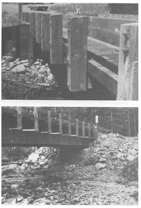
Figure 10-9. - Typical vehicular railing configurations used on timber bridges (continued). (B) Lumber posts attached to steel plates that are bolted through a glulam deck. (C) Lumber posts bolted to a lumber curb with braces attached to a glulam beam.
