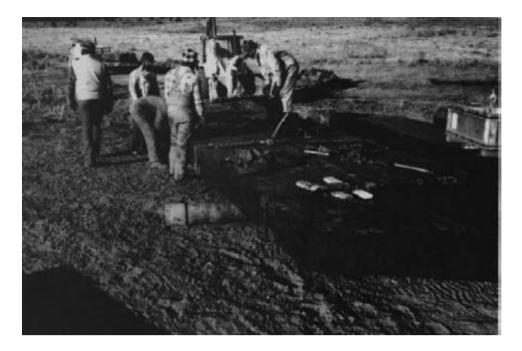
Figure 15-69. - The first two panels of the new bridge are interconnected with steel dowels and pulled together with a come-a-long. Because the crossing was skewed, the doweled panels could not be assembled on the abutments. Assembly was completed adjacent to the site on two well casings to facilitate assembly and lifting.
