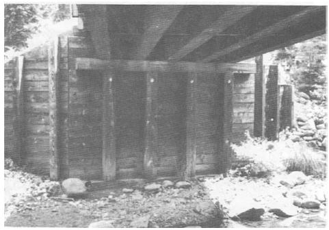
Figure 2-31.- Sawn lumber post abutment.
