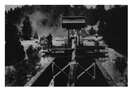
Figure 12-15. - Glulam deck panels are sequentially lifted into place with a backhoe, using C-brackets over the panel ends.
