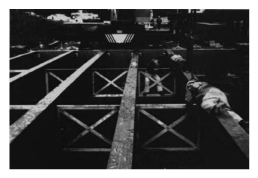
Figure 12-14. - Glulam beams for this bridge are placed from left to right, starting with the outside beam. As the beams are placed in position, bolts are inserted through bearings and steel cross-frames (photo courtesy of Western Wood Structures, Inc.).
