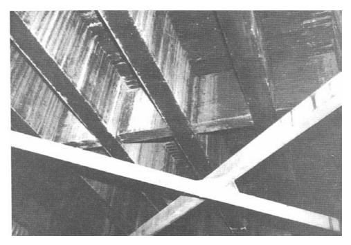
Figure 7-31. - Lumber blocks placed as transverse bracing for sawn lumber beams.
