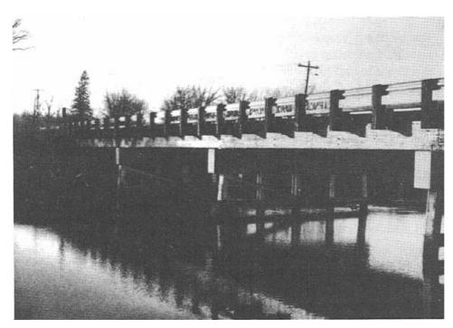
Figure 8-9. - Multiple-span longitudinal nail-laminated lumber deck bridge consisting of a series of simple spans (photo courtesy of Wheeler Consolidated, Inc.).
