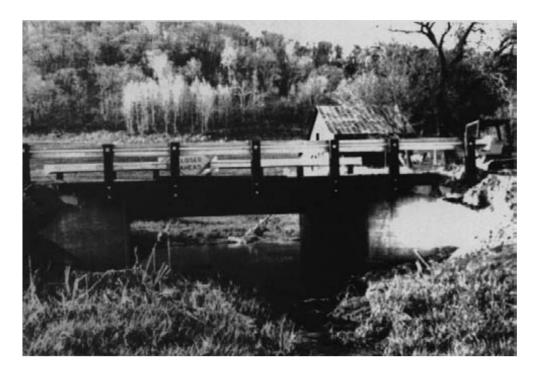
Figure 15-26. - The completed project with widened roadway, ready for paving.
