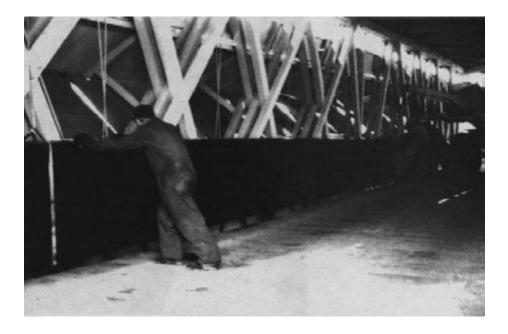
Figure 15-29. - Support for the roadway was obtained by installing two pressure-treated glulam girders inside the existing bridge, one along each side of the roadway.
