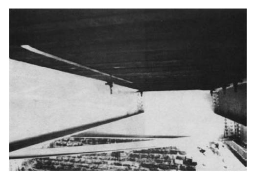
Figure 15-53. - Panels were attached to the stringers with 3/4-inch-diameter by 9-inchlong machine bolts, using a 3/4-inch offset shoe and spring. The offset shoe grips the flange of the stringer, and the compression spring compensates for changes in deck thickness from moisture changes in the timber.
