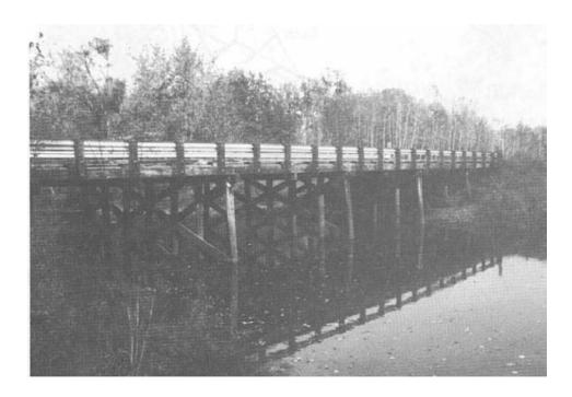
Figure 2-11.- Sawn lumber longitudinal deck bridge. Note the transverse distributor beams attached to the deck underside between bents (photo courtesy of Wheeler Consolidated, Inc.).
