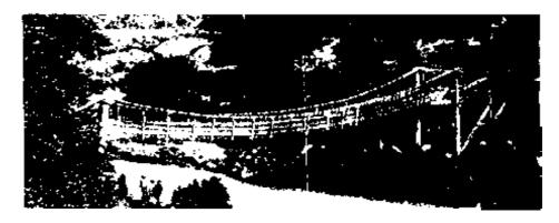
Figure 1-1.—Early highway type of rope bridge. This example is from the island of Java and has an apparent span of approximately 100 feet (photo courtesy of the American Society of Civil Engineers: © 1976. Used by permission).
