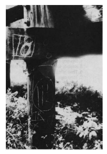
Figure 15-1. - Typical investigative borehole pattern.
