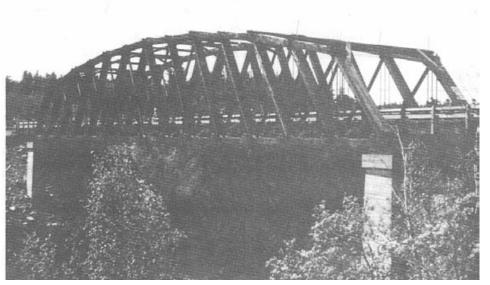
Figure 5-6.- Tension members in bridge applications are most common in trusses. This timber truss, located at Sioux Narrows, Ontario, Canada, spans 210 feet and is reputed to be the longest clear-span timber bridge in the world.
