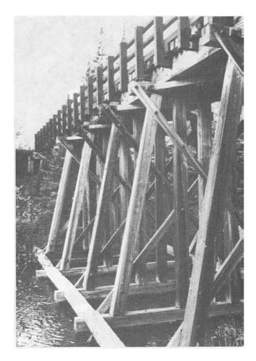
Figure 2-34.- Sawn lumber frame bent.
