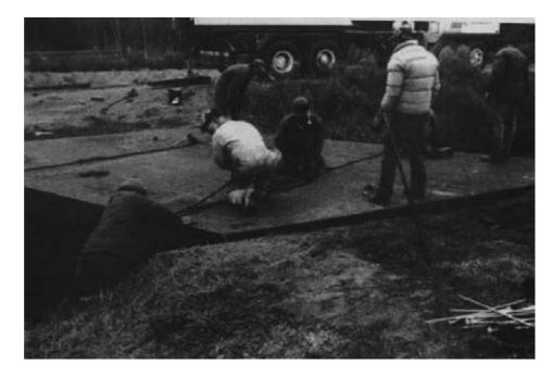
Figure 15-73. - The replacement deck in place.
