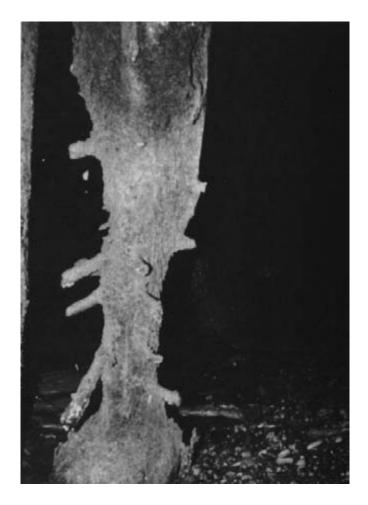
Figure 13-18. - Limnoria damage to a timber pile, evidenced by the characteristic hourglass shape in the tidalzone.
