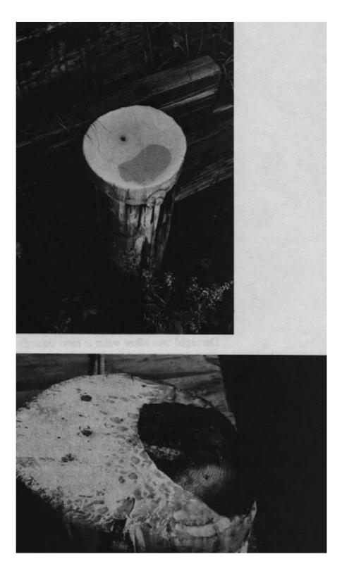
Figure 13-42. - (Top) Damaged metal pile caps allow water to enter, but restrict air circulation and drying. (Bottom) Pile decay is exposed when the damaged cap is removed.
