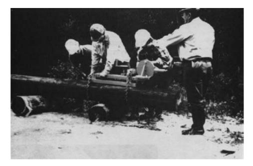
Figure 15-3. - Cutting a replacement pile section using a specially designed pile cutter.
