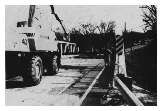
Figure 15-50. - New, prefabricated treated-timber deck panels were placed with a hydraulic excavator. The panels were designed to fit transversely on the stringers and were placed without removing the existing railing.
