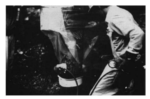
Figure 15-9. - Injection of liquid preservative solution into a timber pile.
