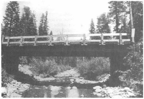
Figure 7-30. - Typical sawn lumber beam bridge with a transverse nail-laminated deck.
