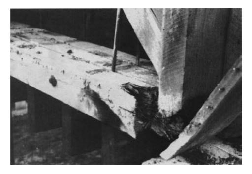
Figure 15-32. - Severe deterioration at each corner of the bridge was one cause of the poor truss alignment. New floorbeams were extended beyond the girders to help support each truss.
