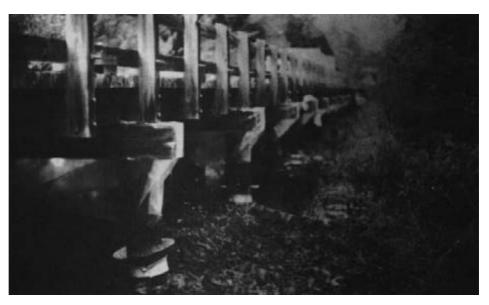
Figure 15-11. - Bridge draping for spillage protection, in place and ready for preservative injection.
