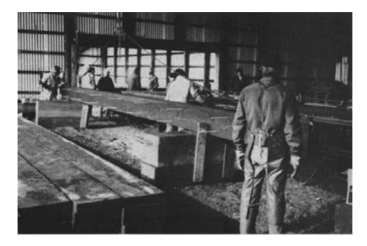
Figure 12-2.- Shop fabrication of timber bridge components, such as these nail-laminated lumber deck panels, is more accurate and more cost effective than field fabrication (photo courtesy of Wheeler Consolidated, Inc.).
