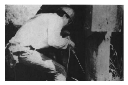
Figure 15-5. - Drilling holes for solid preservative cartridges.
