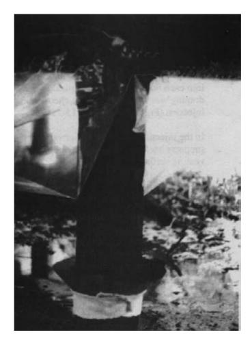
Figure 15-10. - Typical individual cap and pile draping and funnel for protection against leakage of the liquid preservative.
