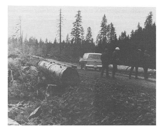
Figure 2-3.- Log beam bridge with a gravel deck. The two large "brow" logs along each side serve to delineate the roadway and function as a type of railing.
