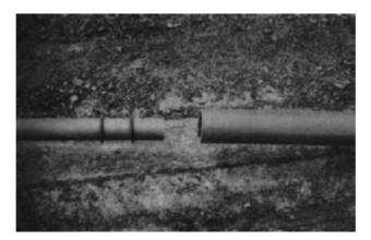
Figure 15-41. - PVC sleeve connection with neoprene O-rings.
