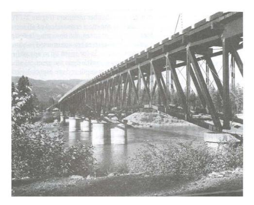
Figure 2-15.- A multiple-span parallel-chord deck truss bridge.
