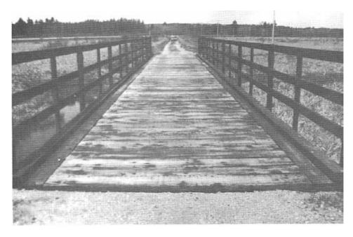
Figure 7-41. - Transverse plank deck on a single-lane, low-volume road (photo courtesy of Wheeler Consolidated, Inc.).
