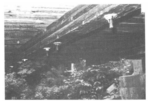
Figure 8-4. - Transverse glulam stiffener beam attached to the underside of a longitudinal glulam deck bridge (photo courtesy of Dave Nordenson, USDA Forest Service).
