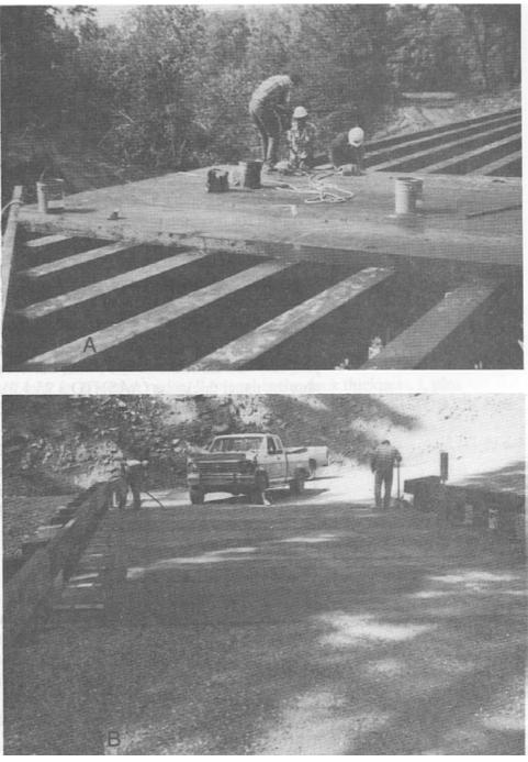
Figure 7-18. - (A) Noninterconnected glulam deck being placed (photo courtesy of LamFab Wood Structures, Inc.). (B) Completed glulam deck is prepared for paving (photo courtesy of Ron Vierra, USDA Forest Service).
