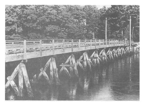
Figure 2-16.- Sewall's bridge is a timber trestle vehicle bridge in York, Maine. The bridge was built in 1933 using the same design features of the original bridge, built in 1761, that it replaced. This bridge became a designated landmark of the American Society of Civil Engineers in 1986 (photo courtesy of the American Society of Civil Engineers; Used by permission).
