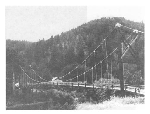
Figure 2-21.- Typical timber suspension bridge designed for vehicle traffic.
