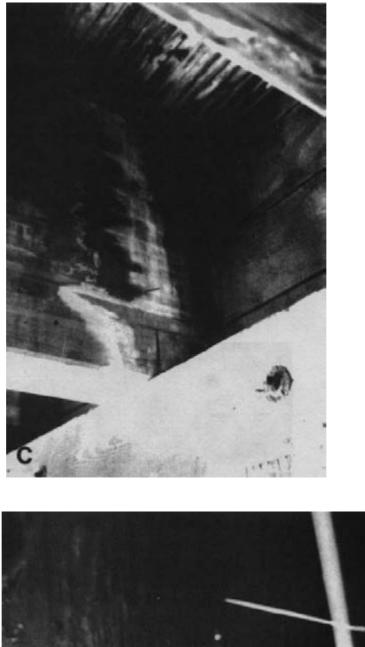
Figure 13-22. - Visual signs of potential deterioration (continued). (C) Water staining. (D) Insect activity (powder posting).
