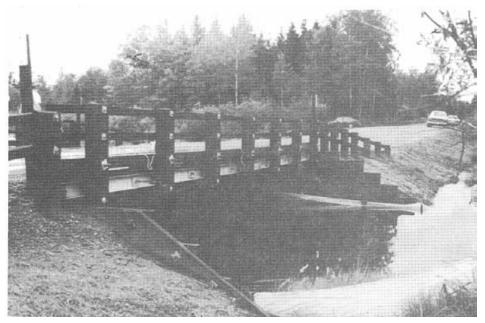
Figure 9-2. – Stress-laminated deck bridge built over Iron River on the Cheguamegon National Forest in 1988.
