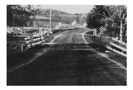
Figure 15-18. - Typical concrete bridge on Pepin County Trunk Highway Z before rehabilitation. The bridges were adequate hydraulically and structurally, but did not meet minimum standards for roadway width.
