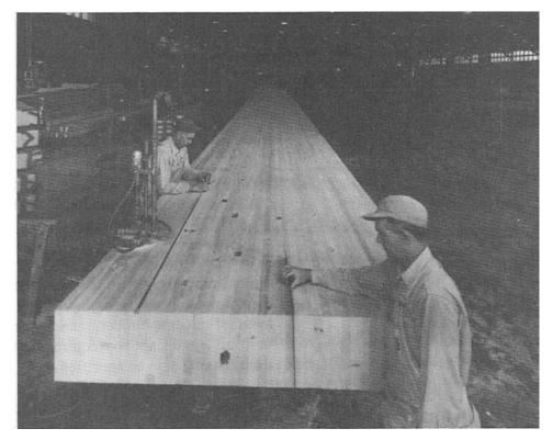
Figure 3-29.-A glulam bridge beam in the final stages of fabrication. The beam, which measures 12-1/4 inches wide, 71-1/2 inches deep and 103 feet long, required 12,800 board feet of structural grade Douglas-fir and 500 pounds of glue.
