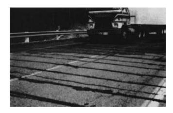
Figure 15-42. - Top prestressing bars installed in grooves cut in the asphalt wearing surface of the North Pagwatchuan River Bridge near Terrace Bay, Ontario.
