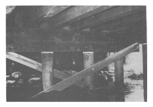
Figure 2-4.- Underside of a sawn lumber beam bridge showing the characteristic close beam spacing. This photo is of the center bent of a two-span crossing, where beams from the two spans overlap at the support.
