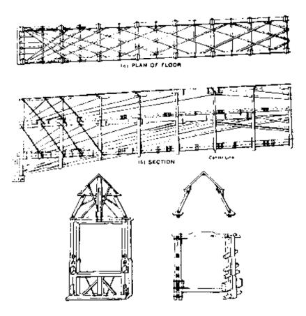
Figure 1-4.-The Schaffhausen Bridge constructed in 1758 over the Rhine River in Switzerland (photo courtesy of the American Society of Civil Engineers; <sup>©</sup> 1976. Used by permission).
