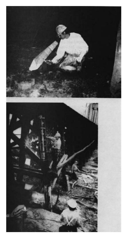
Figure 14-17. - Pile repair using pile restoration techniques (continued). (B) A replacement section is cut, and epoxy gel is applied to the contact surfaces. (C) The replacement section is placed and banded to the existing pile (photos courtesy of Osmose Wood Preserving, Inc.).
