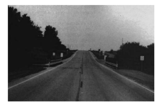
Figure 11-3. - Asphalt pavement wearing surface on a timber bridge deck.
