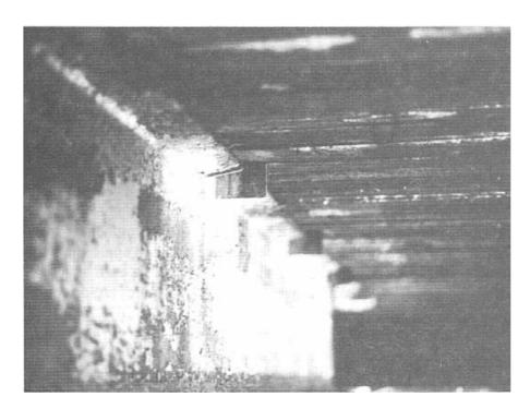
Figure 7-40. - Steel plate deck attachment for nail-laminated lumber decks on steel beams. The thin steel plate is placed over the top beam flange and is nailed to the lumber laminations during deck construction.
