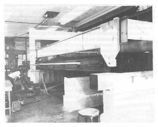
Figure 9-4. - Full-scale experimental stress-laminated deck in the structures laboratory at the University of Wisconsin.
