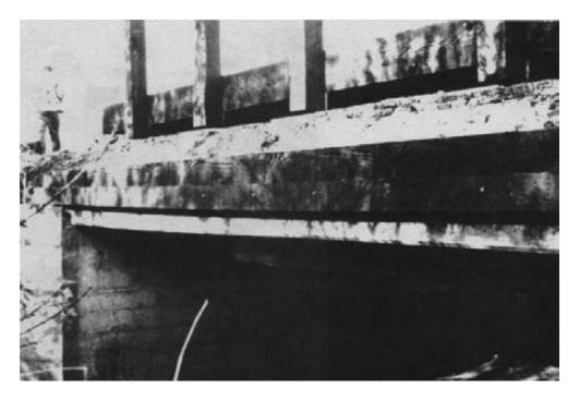
Figure 15-20. - A 4-inch-thick by 14-inch-wide creosote-treated Douglas-fir plank was attached to the edge of the existing concrete deck with galvanized machine bolts and cinch type anchors. The ends of this plank rest on the concrete placed on the wing walls. A 4-inch-thick by 7-inch-wide splice plank was spiked to the bottom half of the plank to form a ship-lap-type joint with the timber deck panel.
