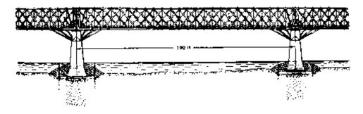
Figure 1-16.- Howe truss built over the Connecticut River at Springfield, Massachusetts, in 1840 (photo courtesy of the American Society of Civil Engineers; <sup>©</sup> 1976. Used by permission).
