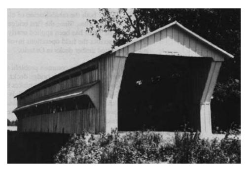
Figure 15-37. - The completed rehabilitation results in a significantly increased load capacity (18 tons), while maintaining the historic bridge's aesthetic appeal.
