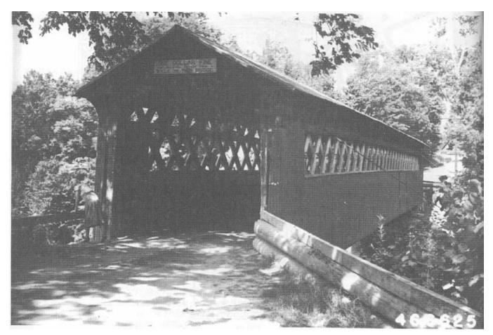
Figure 1-13.-Typical Town lattice truss covered bridge.
