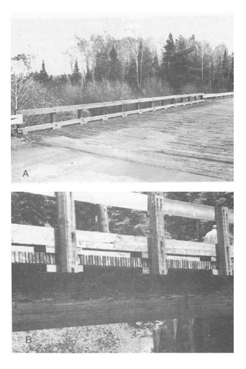
Figure 2-23.- Nail-laminated lumber deck as viewed from (A) the deck top and (B) the deck edge.
