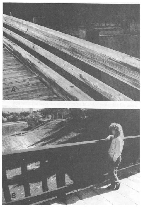
Figure 10-13. - Typical pedestrian/bicycle railing configurations used on timber bridges. (A) Glulam rails mounted on glulam posts. (B) Lumber posts with horizontal rails and vertical pickets.
