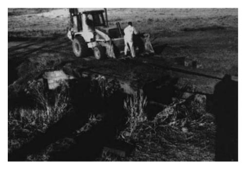
Figure 15-67. - The existing deck was carefully removed in sections to avoid damage to the treated-timber abutment caps.
