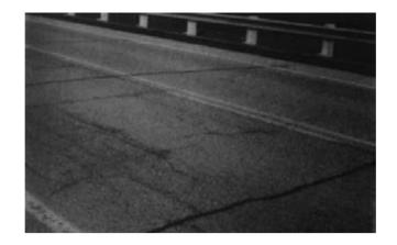
Figure 15-38. - Breakup of asphalt pavement because of delamination of the nail-laminated timber deck.
