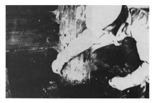
Figure 15-6 - Insertion of solid preservative cartridges into a timber pile. Note the use of rubber safety gloves.
