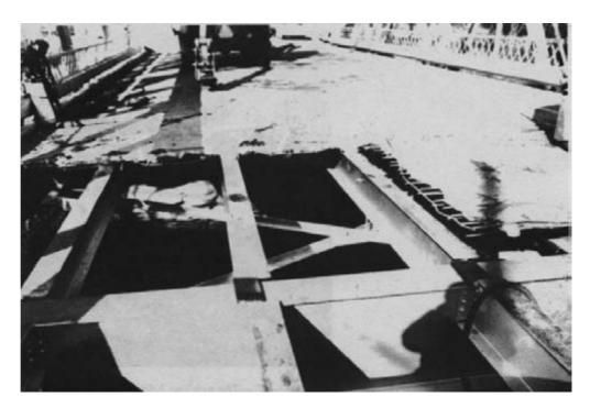
Figure 15-49. - Exposed steel floorbeams and stringers as deck removal proceeds.
