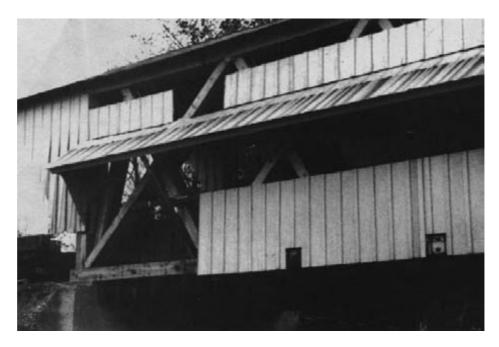
Figure 15-34. - Completed repair of one corner of the bridge, using poplar timbers. Note the closer spacing of the endmost floorbeams to account for the reduced floorbeam load distribution adjacent to the abutment.
