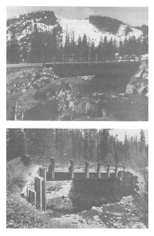
Figure 7-1. - Beam superstructures constructed of (A) glulam timber and (B) sawn lumber.
