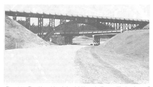
Figure 2-20.- Three-hinge glulam deck arch bridge at the Keystone Wye interchange off U.S. Highway 16, near Mount Rushmore, South Dakota. The arch spans 155 feet and supports a 26-foot-wide roadway (photo courtesy of Wheeler Consolidated, Inc.).
