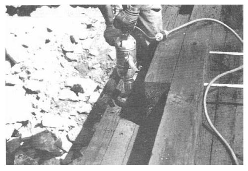
Figure 5-31. - Field-grooving for a split ring connector for a curb-deck attachment. Field fabrication such as this requires field treating with wood preservative, as discussed in Chapter 12 (photo courtesy of Wheeler Consolidated, Inc.).
