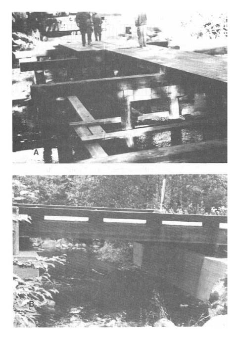
Figure 8-2. - Longitudinal glulam deck bridges. (A) Panel placement during construction of a multiple-span bridge. (B) Typical single-span bridge configuration (photo courtesy of Dave Nordenson, USDA Forest Service).
