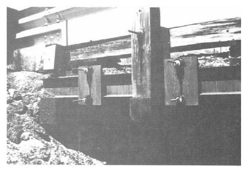
Figure 9-3. - Prestressing rod configuration of the type used on the Hebert Creek Bridge. Rods were placed above and below the existing deck and were anchored to steel plates along the deck edges.
