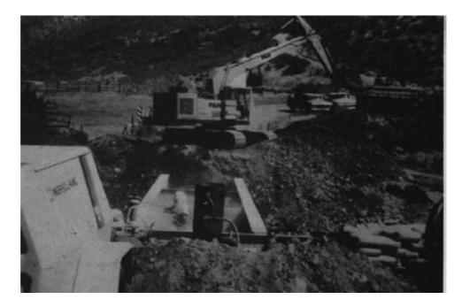
Figure 15-60. - Blast cleaning of the existing steel work in preparation for painting, while a backhoe removes material that was placed for the temporary repair.
