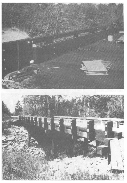
Figure 10-9. - Typical vehicular railing configurations used on timber bridges (continued). (D) Glulam posts and rail with a partial parapet bolted to a glulam deck (photo courtesy of LamFab Wood Structures, inc.). (E) Lumberposts bolted to the lumber curb on a longitudinal nail-laminated lumber deck (photo courtesy of Wheeler Consolidated, Inc.).
