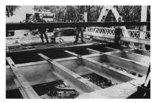
Figure 15-51. - Deck replacement proceeded in stages along the bridge length. After a portion of the concrete was removed, timber deck sections were placed. Steel straps were welded to the ends of the stringers (across floorbeams) to provide continuous support for the timber deck panels.
