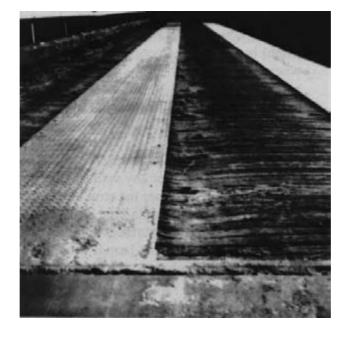
Figure 11-2. - Severe abrasion on a nail-laminated lumber deck caused by vehicles offtracking the partial steel plate wearing surface (photo courtesy of Sakee Poulakidas, USDA Forest Service).
