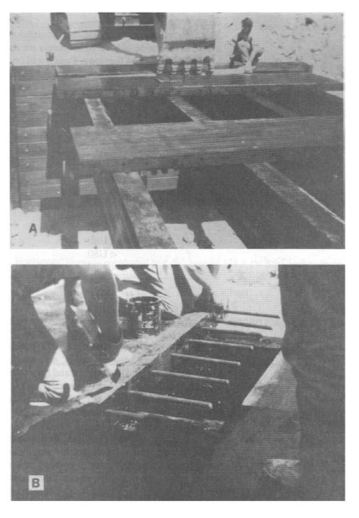
Figure 7-20 - Construction of a doweled glulam deck. The panels are (A) lifted into position and (B) interconnected with steel dowels (photos courtesy of Steve Bunnell, USDA Forest Service).
