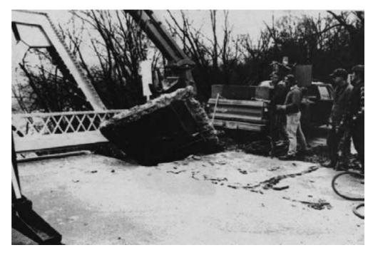
Figure 15-48. - The concrete deck was removed in approximately 5-foot-square sections by the Sauk County High way maintenance crew. The concrete was broken using jackhammers, and reinforcing bats were flame cut. The sections were lifted and loaded on the trucks with a hydraulic excavator.
