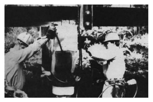
Figure 15-12. - Two-person crew injects liquid wood preservative solution into piles and caps. Note the safety backflow valve on the worker's belt.
