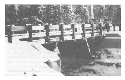
Figure 2-29.- Stress-laminated deck bridge with stress-laminated slant-leg supports, built near Espanola, Ontario, Canada, in 1981. The bridge spans approximately 55 feet and supports two traffic lanes (photo courtesy of the Ontario Ministry of Transportation).
