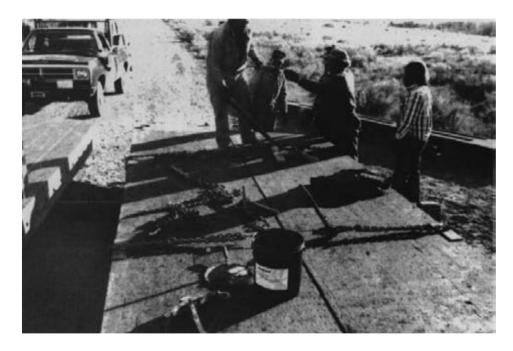
Figure 15-70. - Another view of the first two panels being pulled together. Note the corner protectors under the come-a-long chains and the can of roofing cement on the deck. All panel joints were sealed with the roofing cement before being pulled together.
