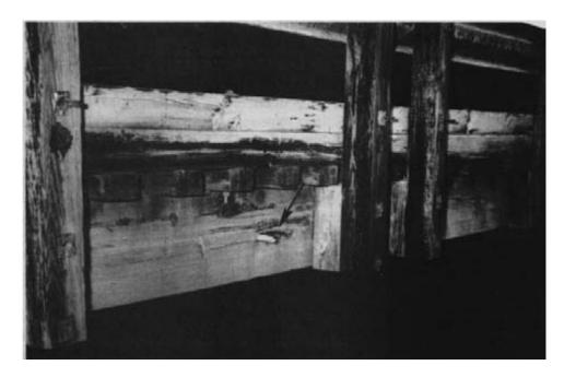
Figure 13-46. - Surface decay on the side of a sawn lumber beam (arrow). Decay in such locations is usually the result of poor preservative penetration of the heartwood.
