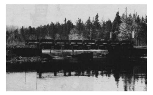
Figure 15-81. - The completed longitudinal stress-laminated deck bridge replaced the existing two-span structure with a single span. The new deck increased load capacity to AASHTO HS 20-44 and included curbs and railing. Remains of the old center support are visible below the replacement structure (photo courtesy of Wheeler Consolidated, Inc.).
