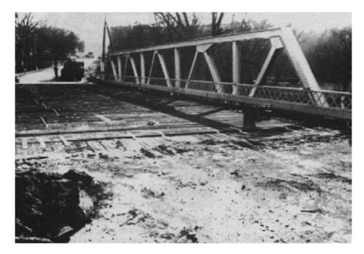
Figure 15-54. - The completed treated-timber deck, before placement of an asphalt-pavement wearing surface.
