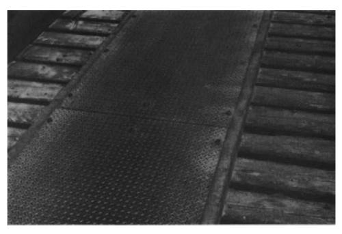
Figure 11-21. - Typical checkered surface pattern on steel running plates.
