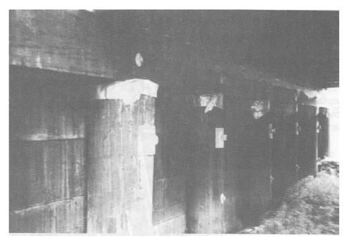
Figure 2-32.- Timber pile abutment.
