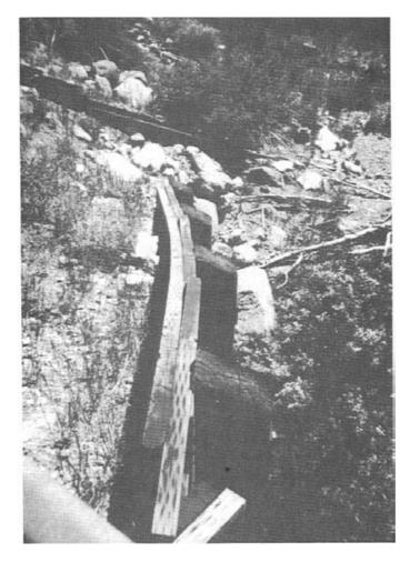
Figure 6-22. - Bulging in an abutment retaining wall caused by earth pressure.
