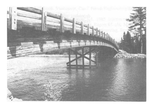
Figure 2-33.- Timber pile bents.
