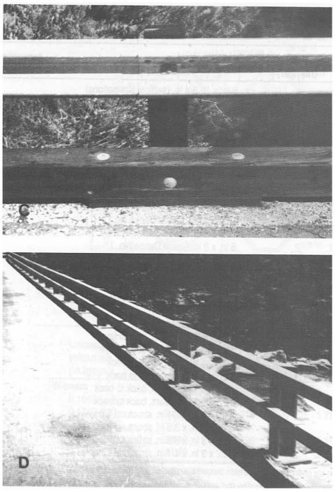
Figure 10-7. - Types of vehicular rails commonly used on timber bridges (continued). (C) Semirigid steel W-beam. (D) Rigid-steel structural tubes.
