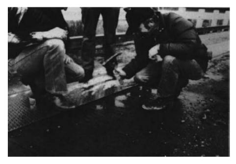
Figure 13-34.- After treating an inspection hole in a bridge deck with liquid wood preservative it is plugged with a treated wood dowel (photo courtesy of Frank Muchmore, USDA Forest Service).
