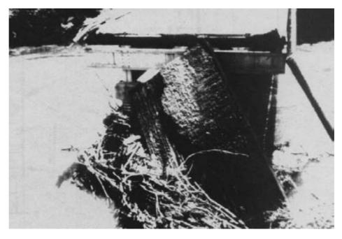
Figure 15-57. - Close-up of the collapsed longitudinal nail-laminated lumber approach span.
