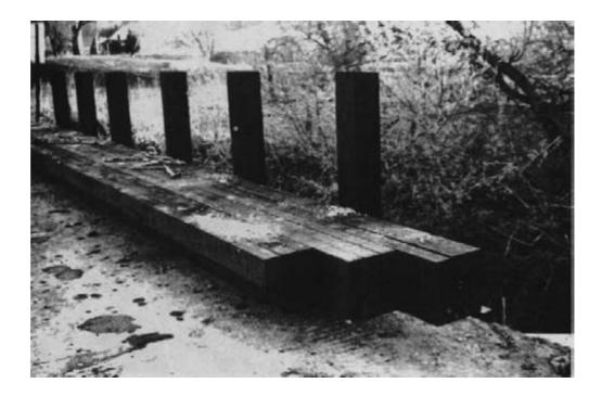
*Figure 15-22. - Rail posts* are attached to the deck panels before the panels are placed on the abutments.
