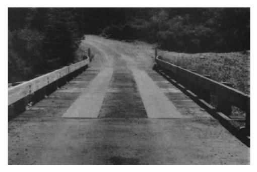
Figure 11-20. - Steel running plate wearing surface on a timber bridge deck.
