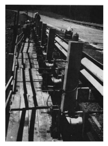
Figure 15-44. - Multijack hydraulic system used at the North Pagwatchuan River Bridge.
