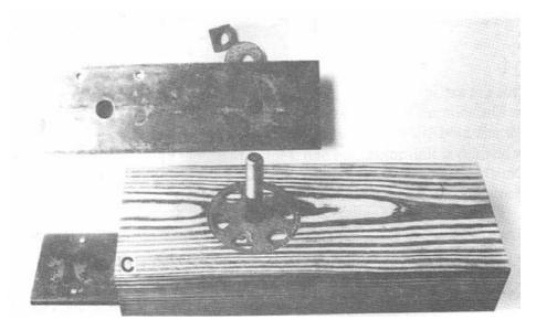
Figure 5-27. - Typical timber connector joints (continued): (C) Shear plate used between wood and steel members.
