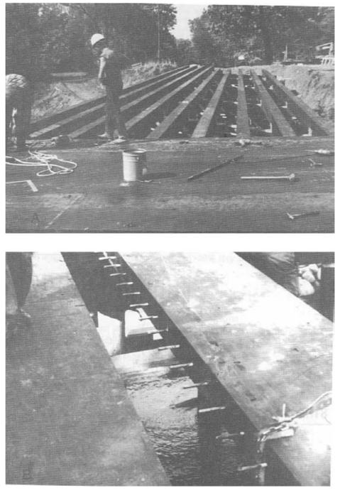
Figure 2-24.- Glued-laminated timber deck in the (A) noninterconnected and (B) doweled configurations.
