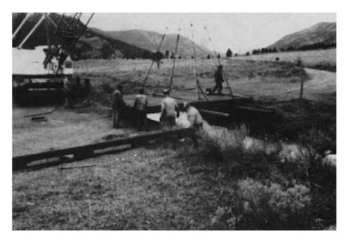
Figure 15-72. - The completed deck, resting on the well casings, is lifted into place on the abutments. Note that the curbs have been preassembled adjacent to site.
