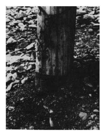
Figure 15-16. - Timber pile after treatment of the soil contact area. The treated portion of the pile was wrapped in waterproof paper to prevent potential soil contamination.
