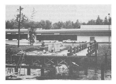
Figure 10-16. - Combination railing posts attached to glulam beams (arrow) through a cutout in the glulam deck (photo courtesy of Western Wood Structures, Inc.).
