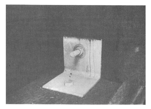
Figure 7-34. - Steel angle bearing attachment for sawn lumber beams.
