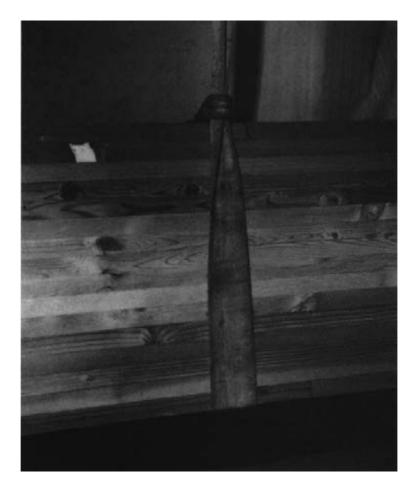
Figure 12-6. - Proper placement of a nylon sling on a glulam beam, with the loop in the sling at the corner of the beam.
