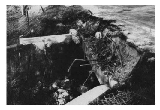
Figure 15-19. - The first step in the rehabilitation was removal of the concrete curb and railing. Next, a concrete seat was poured on the wing walls to support the additional deck width. This bridge also had 2 feet of overburden removed as part of the contract.
