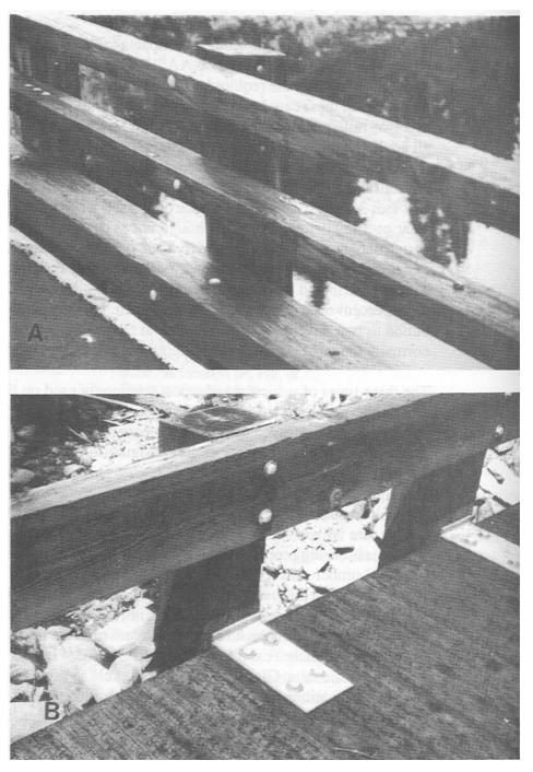
Figure 10-7. - Types of vehicular rails commonly used on timber bridges. (A) Glulam beams. (B) Sawn lumber beam.
