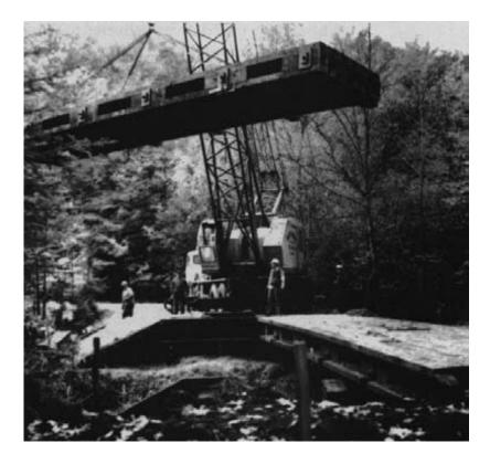
Figure 12-11. - One-half of a stress-laminated parallel-chord bridge is lifted into place by a crane.
