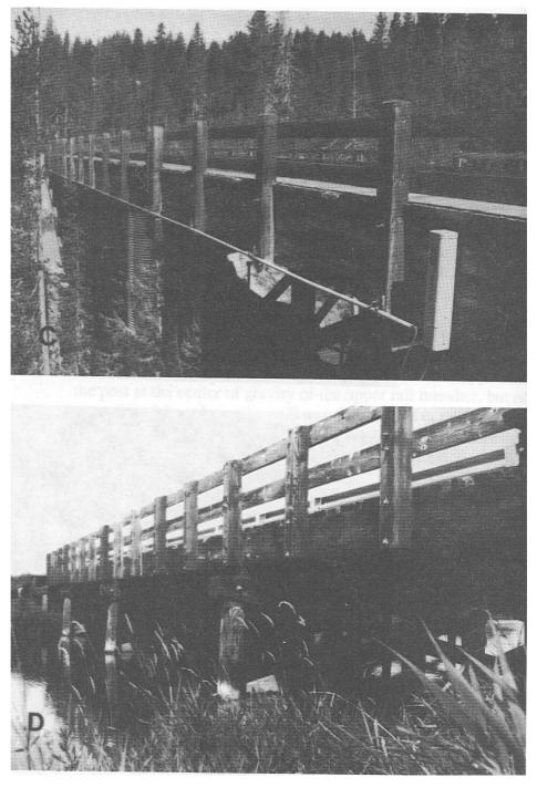
Figure 10-13. - Typical pedestrian/bicycle railing configurations used on timber bridges (continued). (C) Lumber rails on lumber posts that are bolted to a glulam beam. (D) Lumber rails on lumberposts that are bolted to a lumber beam (photo courtesy of Wheeler Consolidated, Inc.).
