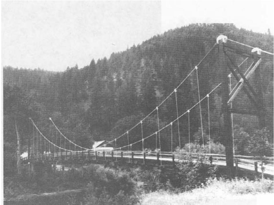
*Figure 2-21.- Typical timber suspension bridge designed for vehicle traffic.*
