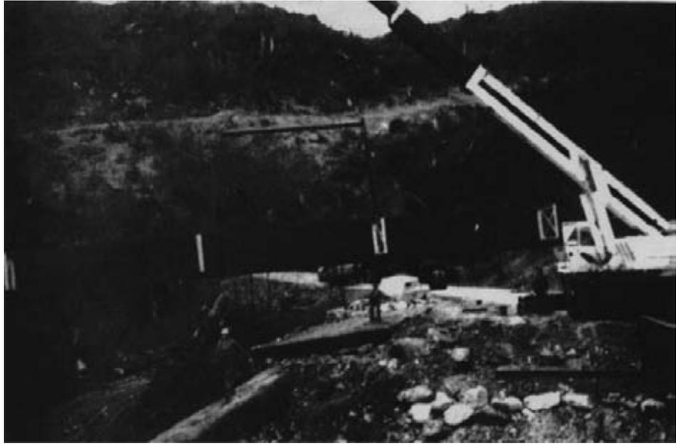
*Figure 12-13. - Glulam beam is lifted into position with steel components in place. Note the use of a spreader beam and nylon straps for lifting (photo courtesy of Western Wood Structures, Inc.).*
