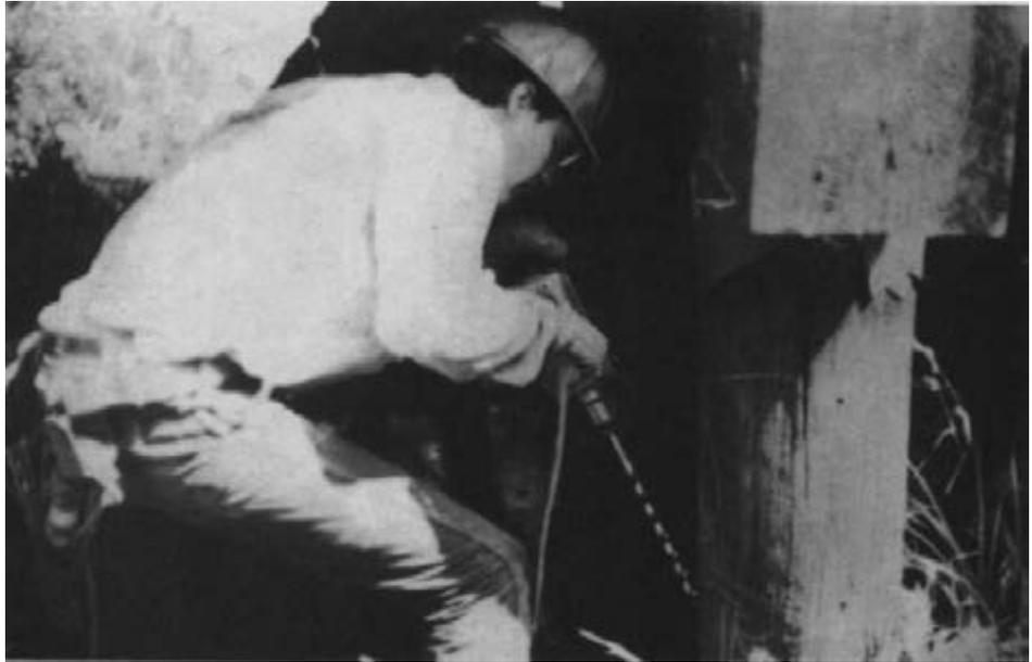
*Figure 15-5. - Drilling holes for solid preservative cartridges.*
