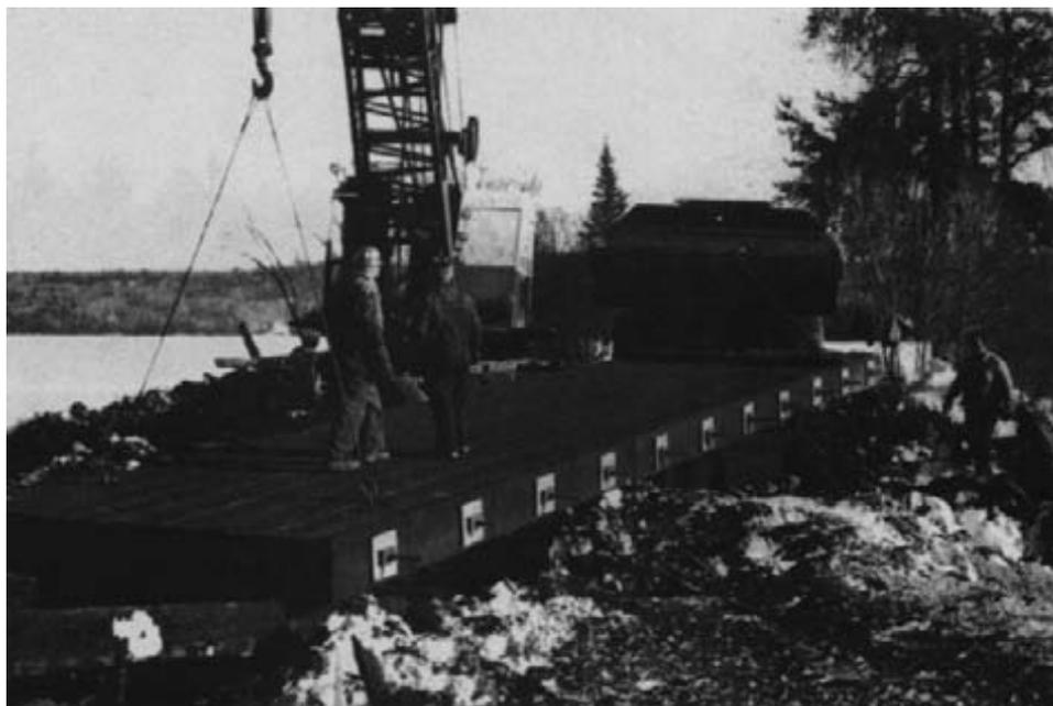
*Figure 15-79. - One of the prefabricated, prestressed, bridge deck panels is lifted into position on the treated-timber crib abutments.*
