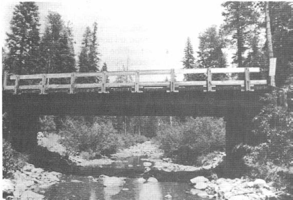
*Figure 7-30. - Typical sawn lumber beam bridge with a transverse nail-laminated deck.*
