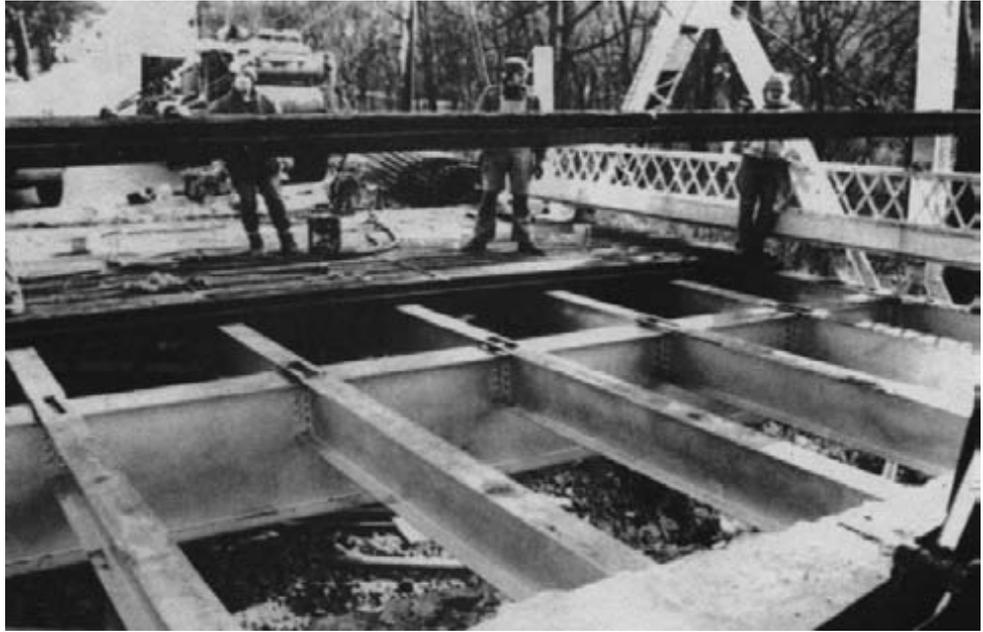
*Figure 15-51. - Deck replacement proceeded in stages along the bridge length. After a portion of the concrete was removed, timber deck sections were placed. Steel straps were welded to the ends of the stringers (across floorbeams) to provide continuous support for the timber deck panels.*
