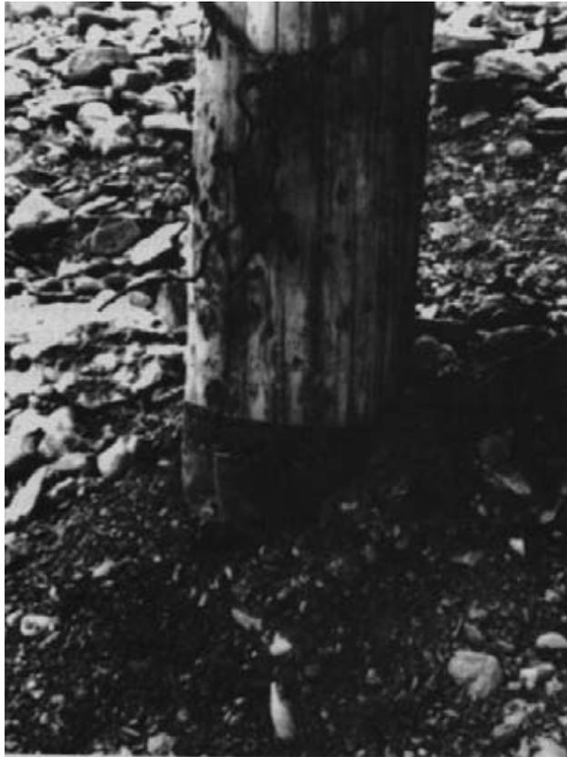
*Figure 15-16. - Timber pile after treatment of the soil contact area. The treated portion of the pile was wrapped in waterproof paper to prevent potential soil contamination.*
