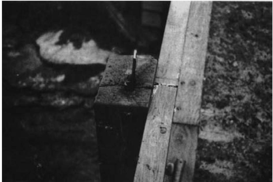
*Figure 13-37. - Decay in the end grain of a timber rail post (photo courtesy of Duane Yager, USDA Forest Service).*
