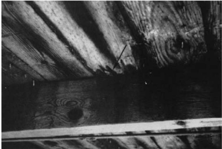
*Figure 13-47. - Decay on the underside of a spike-attached lumber plank deck at the deck-beam interface (arrow).*
