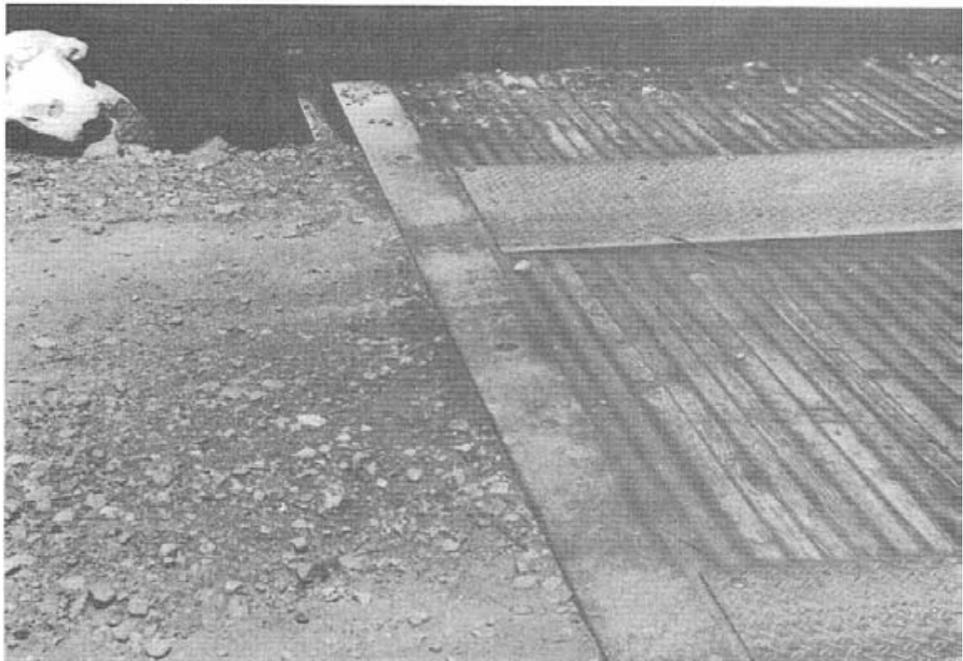
*Figure 7-29. - Steel nosing angle placed across an unpaved deck to reduce damage from vehicle impact and abrasion.*
