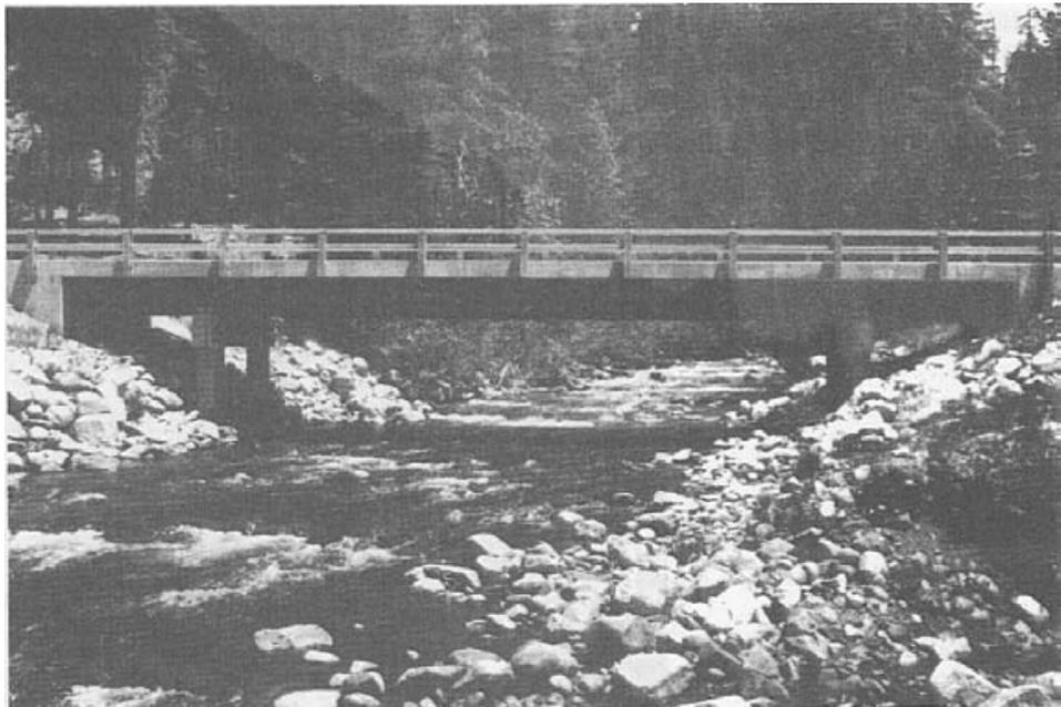
Figure 2-26.- Composite glulam-concrete T-beam bridge located in northern California. Although numerous bridges of this type have been built, they are not common.
