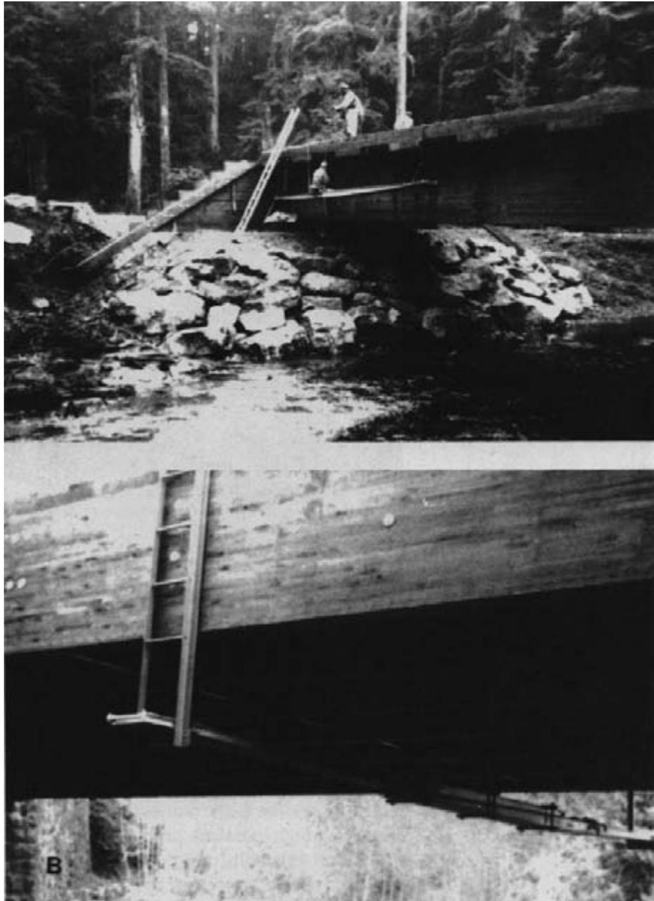
Figure 12-12. - Typical scaffolding configurations for accessing the underside of a glulam beam bridge. (A) Along the deck overhang (photo courtesy of Tim Chittenden, USDA Forest Service). (B) Between beams (photo courtesy of Western Wood Structures, Inc.).
