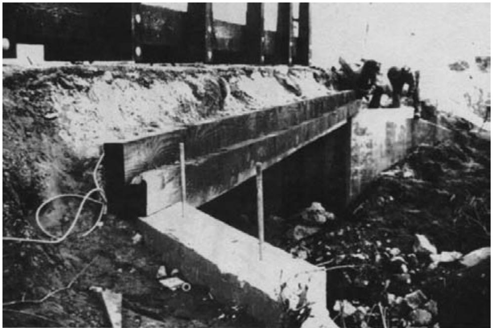
*Figure 15-21. - Anchor bolts are placed in the concrete wingwalls that match predrilled holes in the timber deck panels.*
