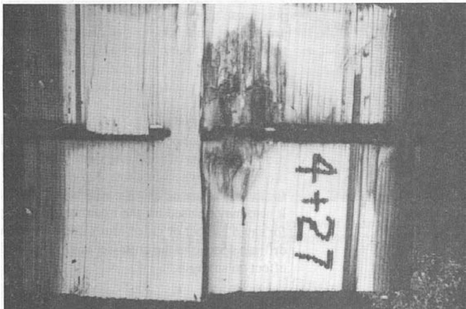
*Figure 4-4.- Decay can originate in field-bored holes that are made after the wood is treated with preservatives. In this member, a hole drilled after treatment exposed untreated wood and eventually led to decay at the center of the member (the horizontal split across the bolt hole was made as the member was removed). Preboring holes prior to pressure treatment can prevent this damage.*
