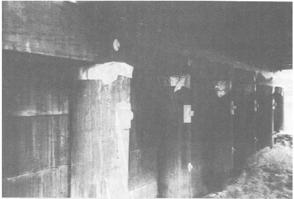
*Figure 2-32.- Timber pile abutment.*
