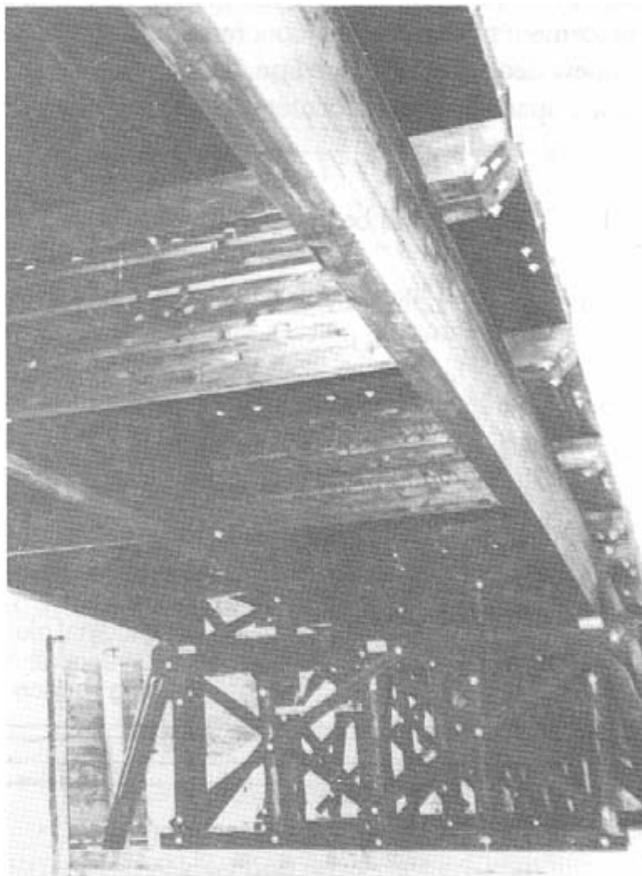
Figure 8-19. - Longitudinal glulam deck on transverse glulam floorbeams.
