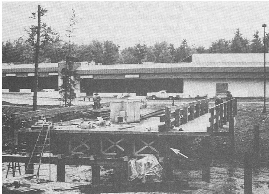
*Figure 10-16. - Combination railing posts attached to glulam beams (arrow) through a cutout in the glulam deck (photo courtesy of Western Wood Structures, Inc.).*
