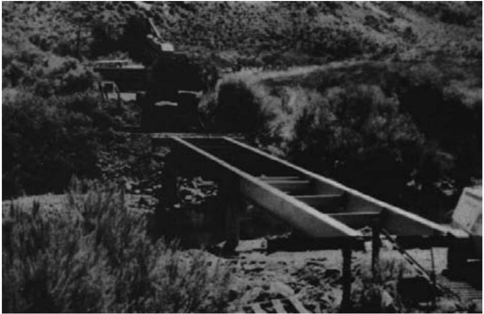
*Figure 15-62. - A portion of the final paint coat has been applied to the steel and the new treated-timber abutments are in-place. The backhoe is positioned to lift the longitudinal glulam panels for the far side approach span.*
