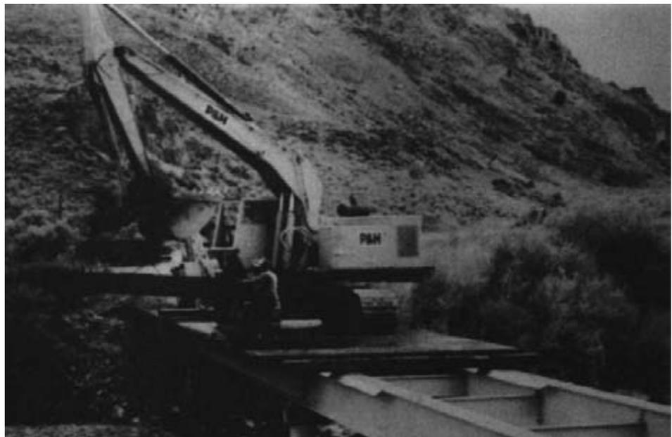
*Figure 15-63. - Transverse glulam deck panels are lifted into place.*
