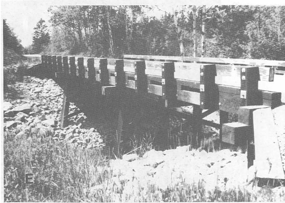
Figure 10-9. - Typical vehicular railing configurations used on timber bridges (continued). (D) Glulam posts and rail with a partial parapet bolted to a glulam deck (photo courtesy of LamFab Wood Structures, inc.). (E) Lumberposts bolted to the lumber curb on a longitudinal nail-laminated lumber deck (photo courtesy of Wheeler Consolidated, Inc.).
