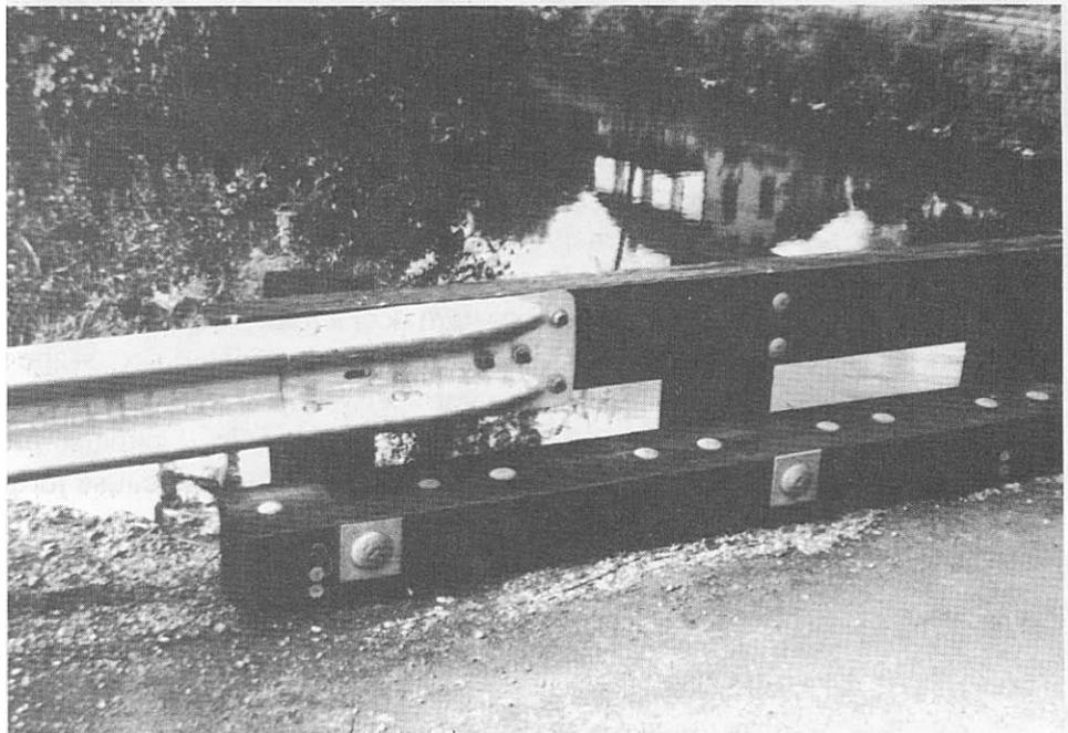
*Figure 10-8. - Standard rail transition between a glulam bridge rail and a steel W-beam approach rail.*
