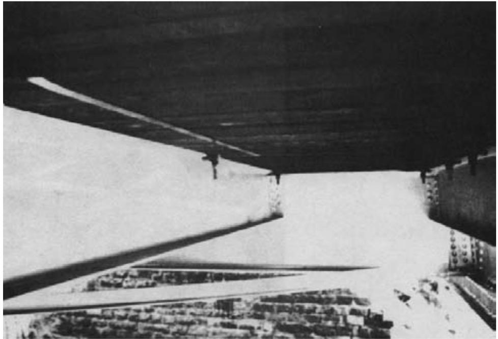
*Figure 15-53. - Panels were attached to the stringers with 3/4-inch-diameter by 9-inch-long machine bolts, using a 3/4-inch offset shoe and spring. The offset shoe grips the flange of the stringer, and the compression spring compensates for changes in deck thickness from moisture changes in the timber.*
