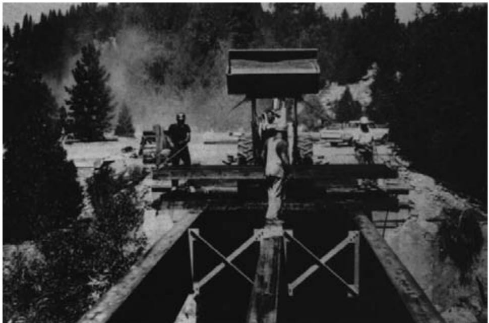
*Figure 12-15. - Glulam deck panels are sequentially lifted into place with a backhoe, using C-brackets over the panel ends.*
