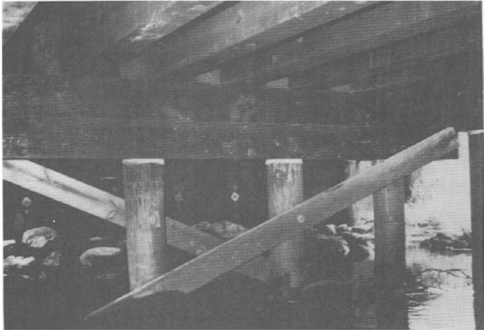
*Figure 2-4.- Underside of a sawn lumber beam bridge showing the characteristic close beam spacing. This photo is of the center bent of a two-span crossing, where beams from the two spans overlap at the support.*
