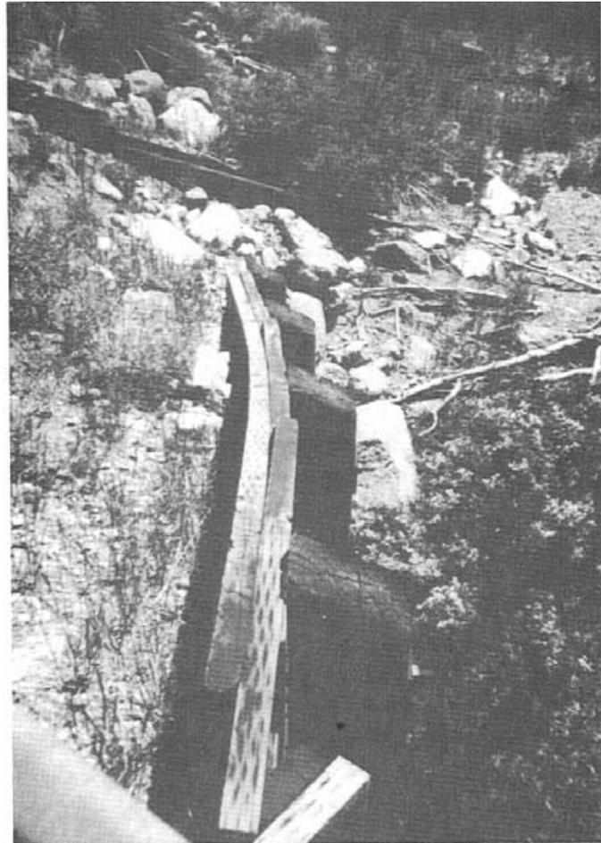
Figure 6-22. - Bulging in an abutment retaining wall caused by earth pressure.
