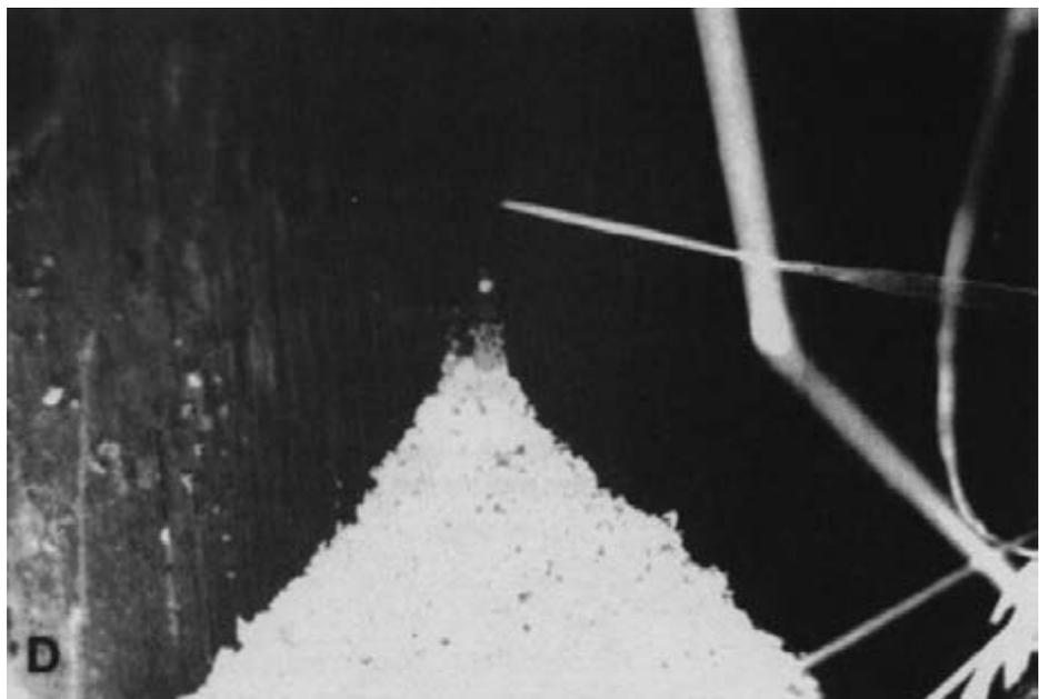
*Figure 13-22. - Visual signs of potential deterioration (continued). (C) Water staining. (D) Insect activity (powder posting).*
