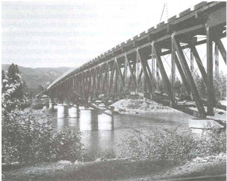
*Figure 2-15.- A multiple-span parallel-chord deck truss bridge.*
