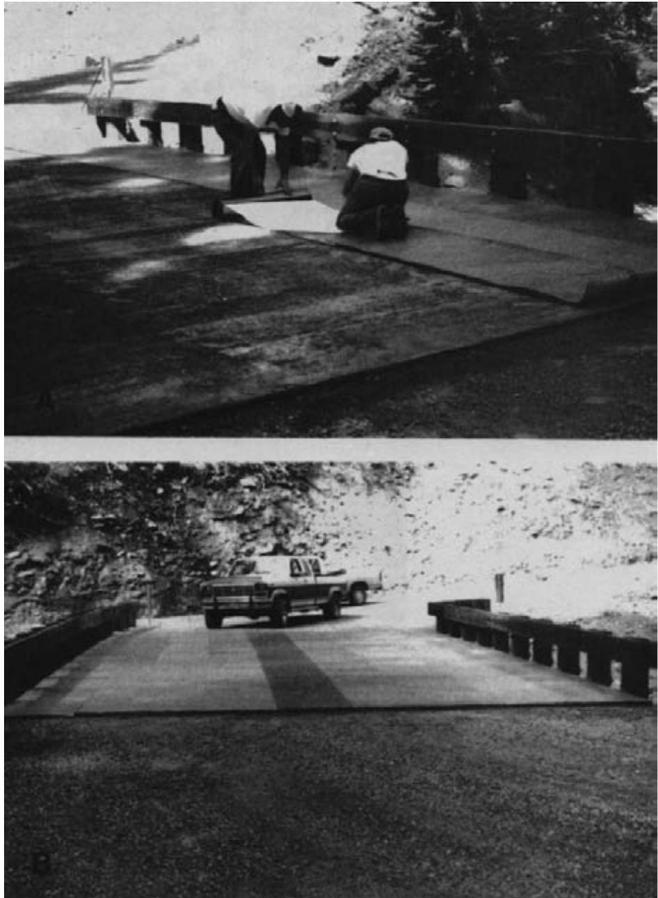
*Figure 11-7. - Asphalt paving sequence on a glulam bridge deck using impregnated geotextile fabric. (A) Geotextile fabric is roiled longitudinally over the cleaned deck (note that the backing paper on the asphalt side of the fabric is removed as the fabric is rolled). (B) Completed fabric placement.*
