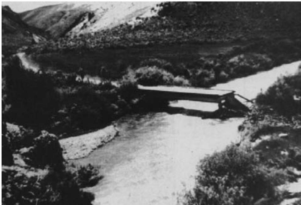
*Figure 15-56. - Collapsed span and breached approaches of the existing bridge.*
