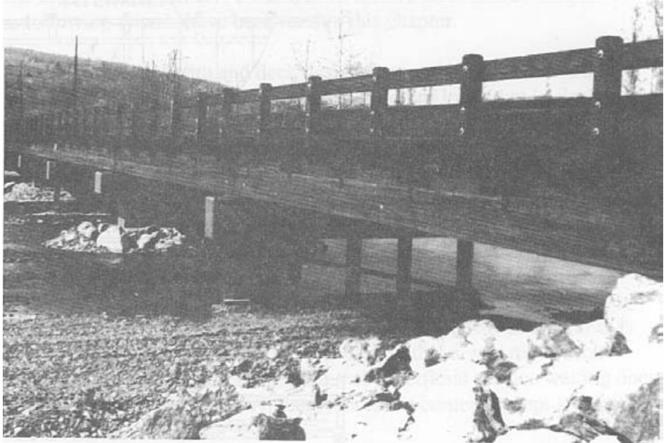
*Figure 7-3.- Glulam beam bridge, 290 feet long in Tioga County, New York. This bridge was completely prefabricated in standardized components that were bolted together at the project site (photo courtesy of Weyerhaeuser Co.).*
